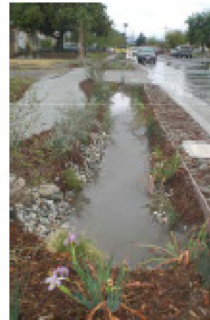
Stormwater flows through a curb inlet into a bioswale on Elmer Street. The water infiltrates into the soil within a day, preventing breeding mosquitoes.
