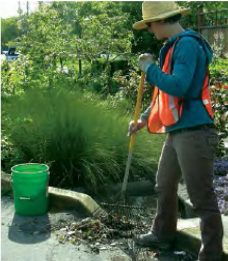
Figure 1. A worker removes sediment and debris from a curb-cut in a stormwater bump-out along a street in Portland, Oregon.
