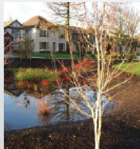
This bioswale pond in Wilsonville, Oregon collects runoff from the rooftops, sidewalks and yards. The pond offers valuable aesthetic and wildlife habitat benefits while also reducing stormwater control costs.
