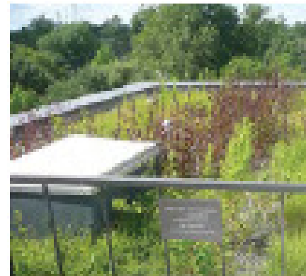
A green roof, such as this one at Sidwell Friends School in Washington, D.C., absorbs rain water, reduces energy costs, and provides green space and wildlife benefits in an urban area.
