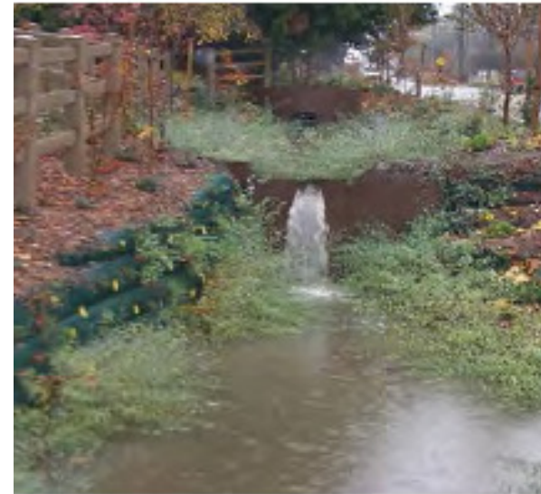
A stair-stepped pool slows runoff in Seattle's NW 110 th Cascade project.
