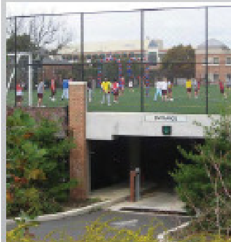
The roof of this Washington, D.C. parking garage doubles as a school athletic field, reducing runoff and offering usable open space.
