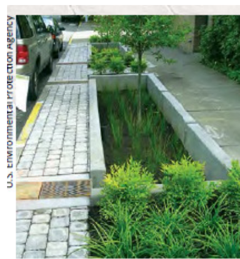
Figure 3. This stormwater planter is one of a suite of dispersed stormwater management practices that Portland, Oregon, city employees help to manage.
