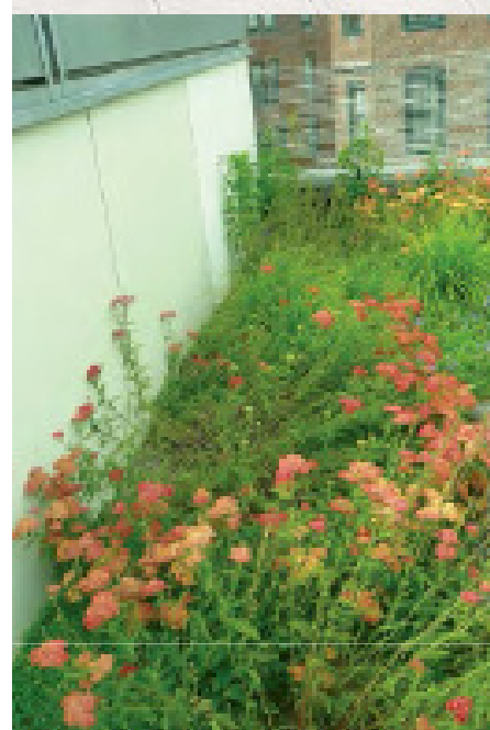
Developers of Philadelphia's Thin Flats condominiums added green roofs that capture rain water and provide private green space, complete with rooftop patios, for each unit.
